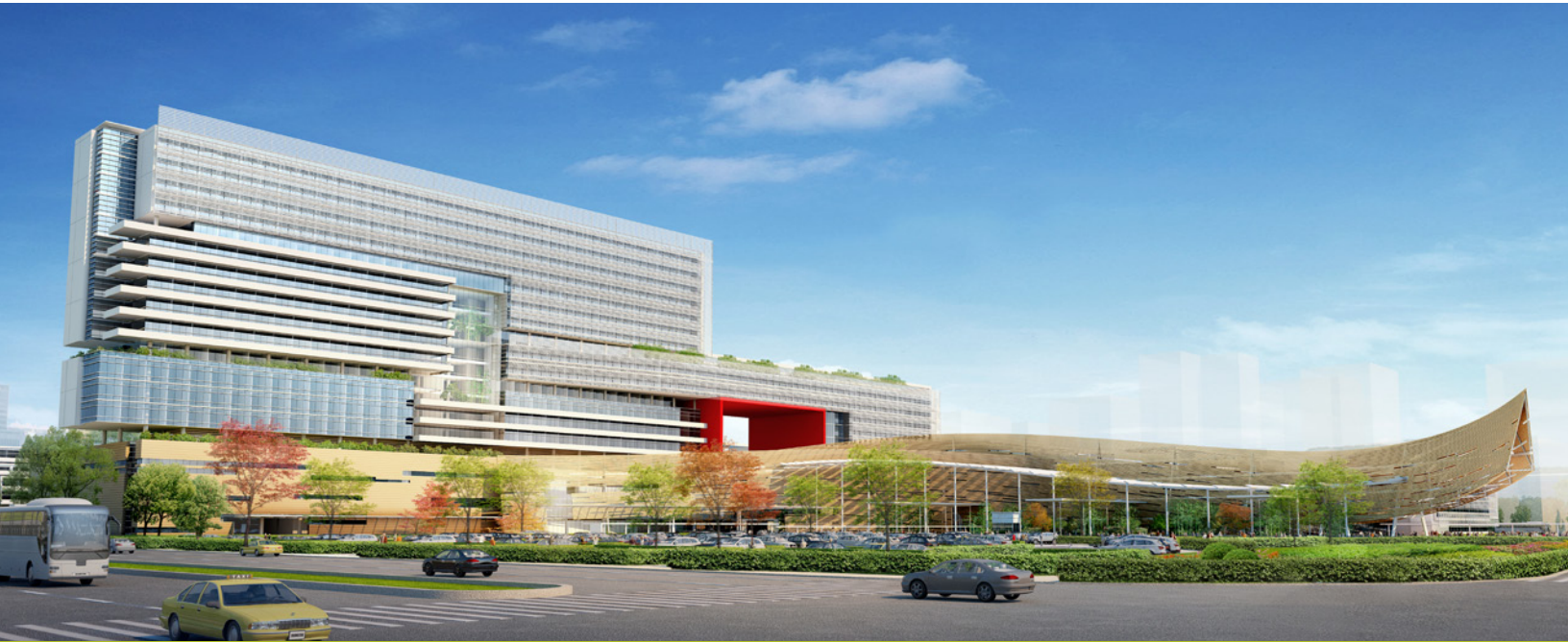
The First People's Hospital, Shunde District, China
