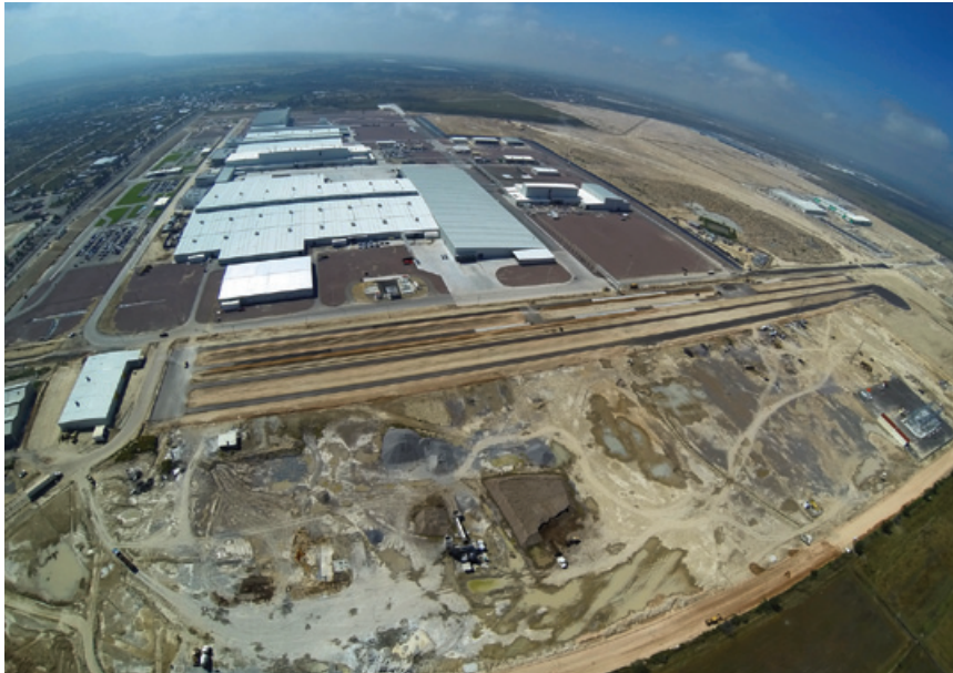
HOT SPOT A recently completed auto assembly facility for Nissan in Mexico, which has plans to expand.
