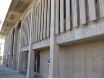
▲ View looking north at existing Hilb Building west elevation
