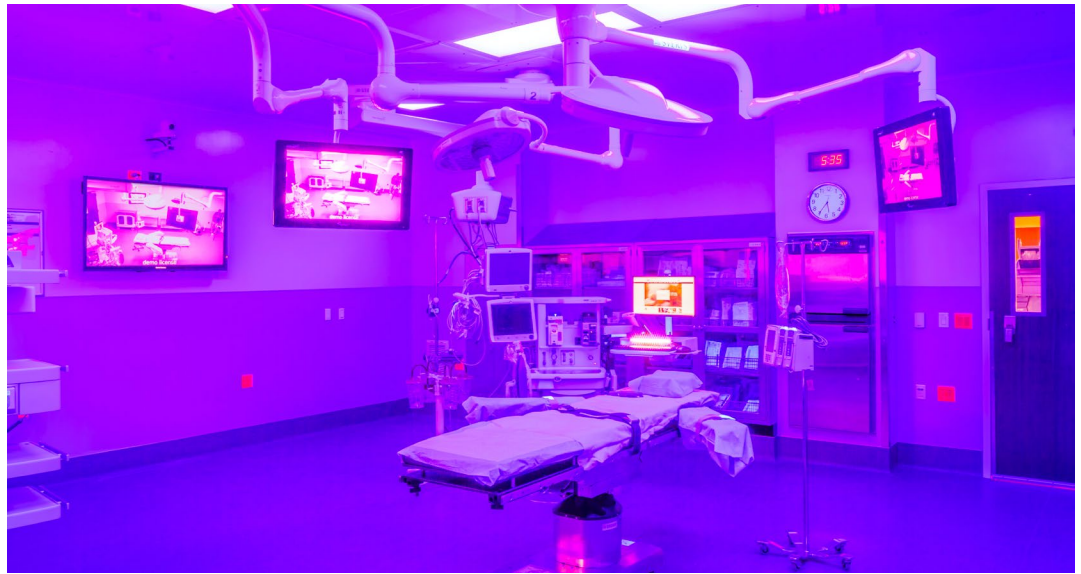
Narrow spectrum lighting for infection control, Henderson Hospital, Henderson, Nev.
